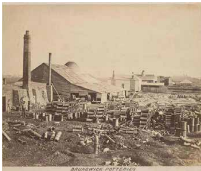
Figure 77: Alfred Cornwell's Pottery, corner of Phoenix and Albert Streets, c.1866, showing the pipes produced at his works. Source: Pictures Collection, State Library of Victoria.
