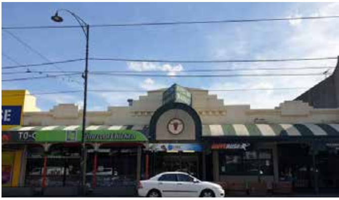
Figure 98: Coburg Market. Source: Extent Heritage Pty Ltd, 2020.
