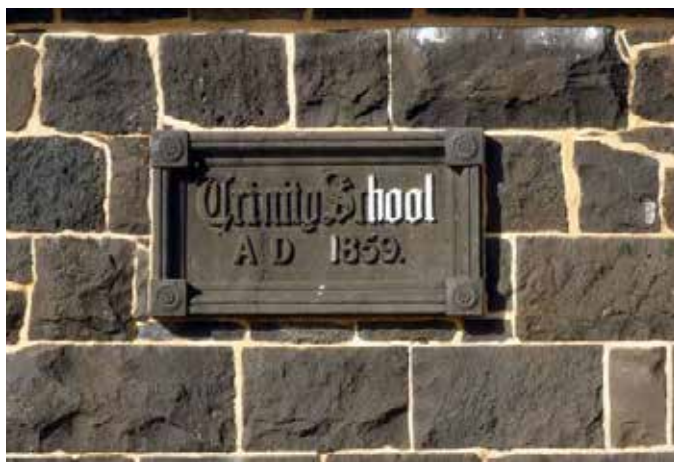
Figure 110: Foundation stone in the bluestone fabric of the Anglican school built in 1859 on Sydney Road, Coburg. Photograph by C Wilmsen, May 2010. Source: Moreland City Council.
