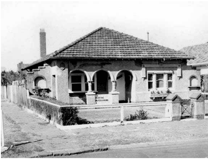
Figure 58: An example of the Spanish Mission style built in c.1938 at 16 Budds Street, Coburg. Source: Coburg Historical Society and Picture Victoria.
