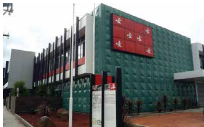
Figure 91: The Craig and Seeley Administration Building after restoration in 2008. The enamel finishes on the exterior remain in excellent condition, a testament to the durability of Craig and Seeley's well-known 'Chef' brand kitchen stoves. Source: Moreland City Council.
