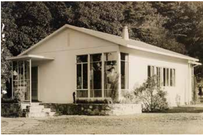
Figure 62: Beaufort Home, on display in the Treasury Gardens, Melbourne in 1946, Volume 5: Beaufort Home construction photographs / Arthur Baldwinson collection. Source: Mitchell Library, State Library of New South Wales.
