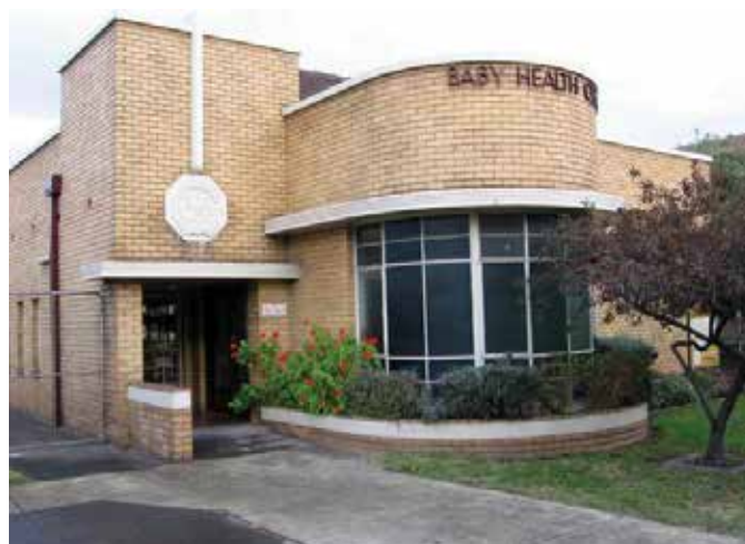
Figure 116: Baby Health Centre in Lygon Street, Brunswick East, which opened in 1939. Photograph by Moreland City Council Activity Centres Team, May 2006. Source: Moreland City Council.
