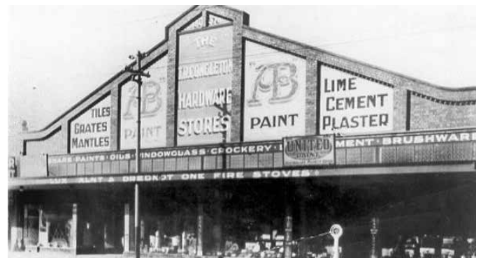
Figure 100: Congleton's Hardware Store, 376-380 Sydney Road, Coburg. Source: Coburg Historical Society and Picture Victoria.
