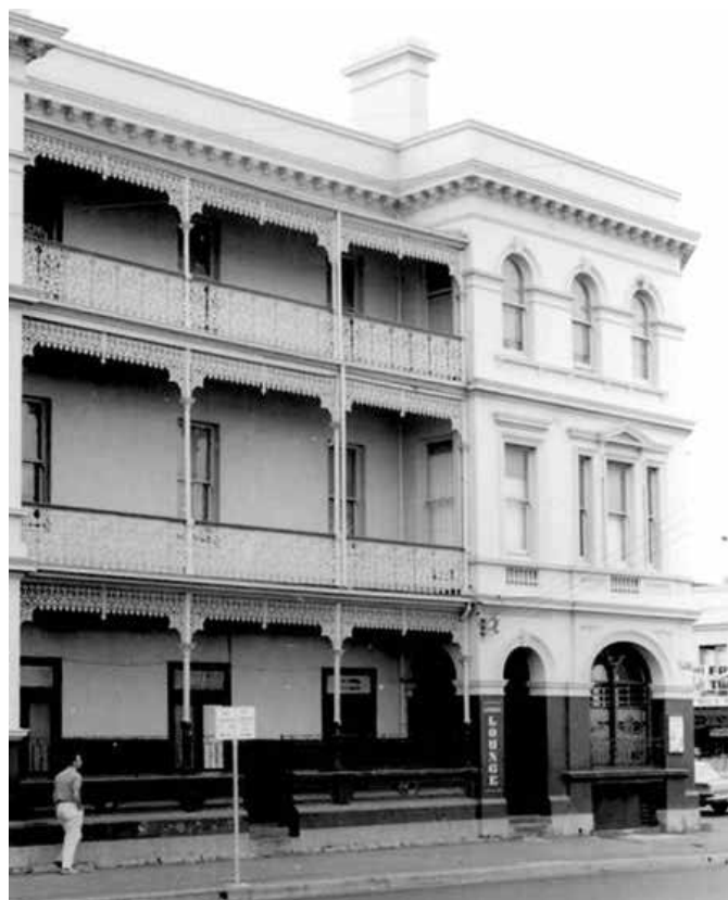
Figure 121: The grand three-storey Lomond Hotel, at 225–231 Nicholson Street (corner Blyth Street), Brunswick East. In 2009 it operates as an unpretentious pub providing live music and old-style counter meals. Photograph by John Collins, 1964. Source: J.T. Collins Collection, Pictures Collection, State Library of Victoria.
