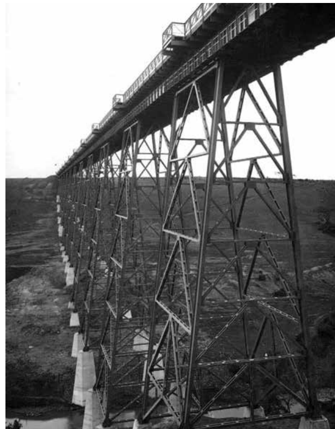
Figure 24: Albion to Broadmeadows Goods Line, Glenroy Viaduct, June 1929. Photograph by Wilfred Chapman. Source: Pictures Collection, State Library of Victoria.
