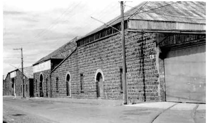
Figure 33: Melville’s Grainstore, Colebrook Street, Brunswick, with rail siding. Photograph by John Collins, January 1982. Source: J.T. Collins Collection, Pictures Collection, State Library of Victoria.
